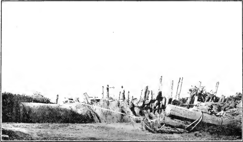
FIG. 9.—FINAL CLOSURE FROM BELOW HYDRAULIC-FILL DAM, HANLON HEADING, SEPTEMBER 20TH, 1915.
